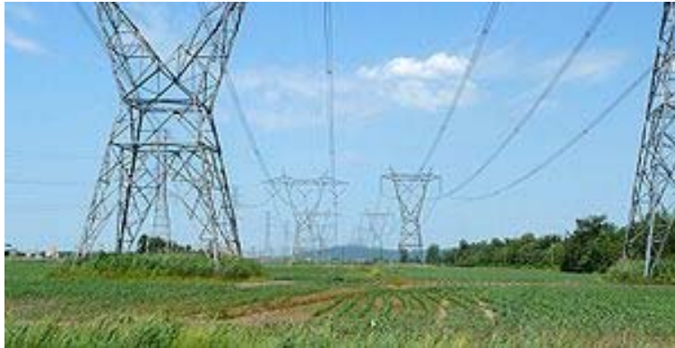
Long power transmission lines
