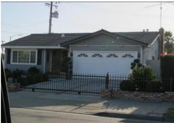
**Figure 24 Average-Sloped Gable Roof**
