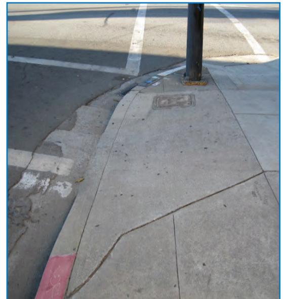
Figure 4.20 Example of a curb cut. The steep, narrow, and cracked sidewalk ramp at the corner of 15th Street and East Santa Clara Street.
