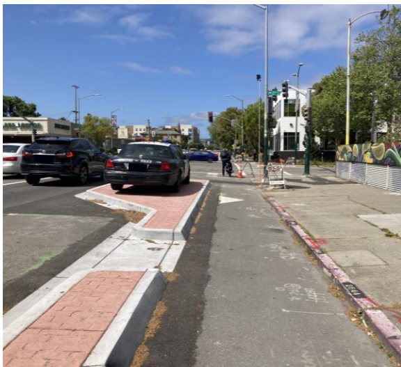
Figure 2.10: Oakland Police parked on the bike lane separator, obstructing the view of cyclists at the corner and driveway interaction.
