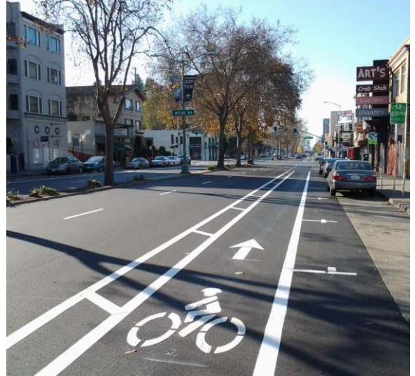
Figure ES.2: Buffered Class II Bike Lane on Broadway in Oakland.
