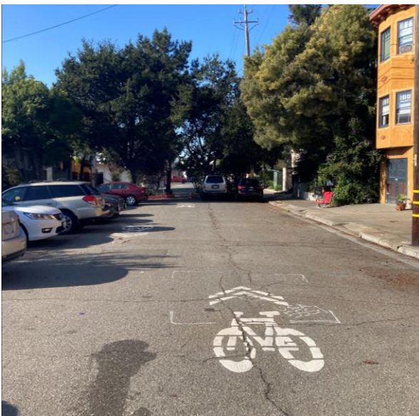
Figure ES.3: Class III Bike Route with sharrow and traffic diverter on 55 th Street in Oakland.
