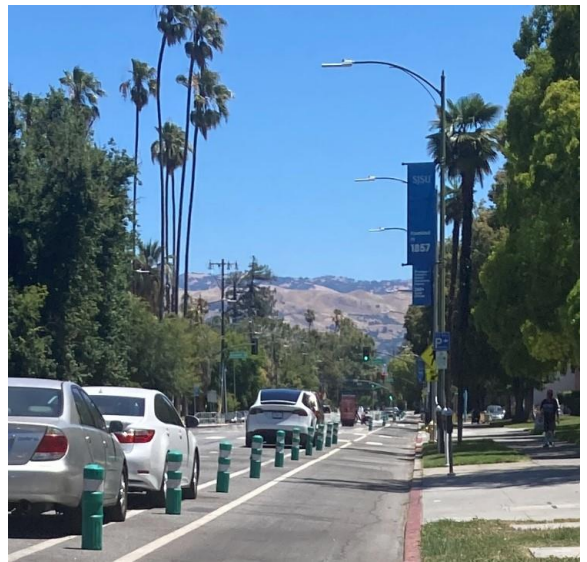
Figure ES.4: Class IV Protected Bikeway on San Fernando Street in San José.
